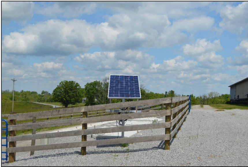
A solar powered pump installed in a water harvesting system.
