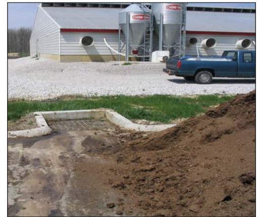
Figure 3. Mortality composting runoff entering drain to travel to existing lagoon.
