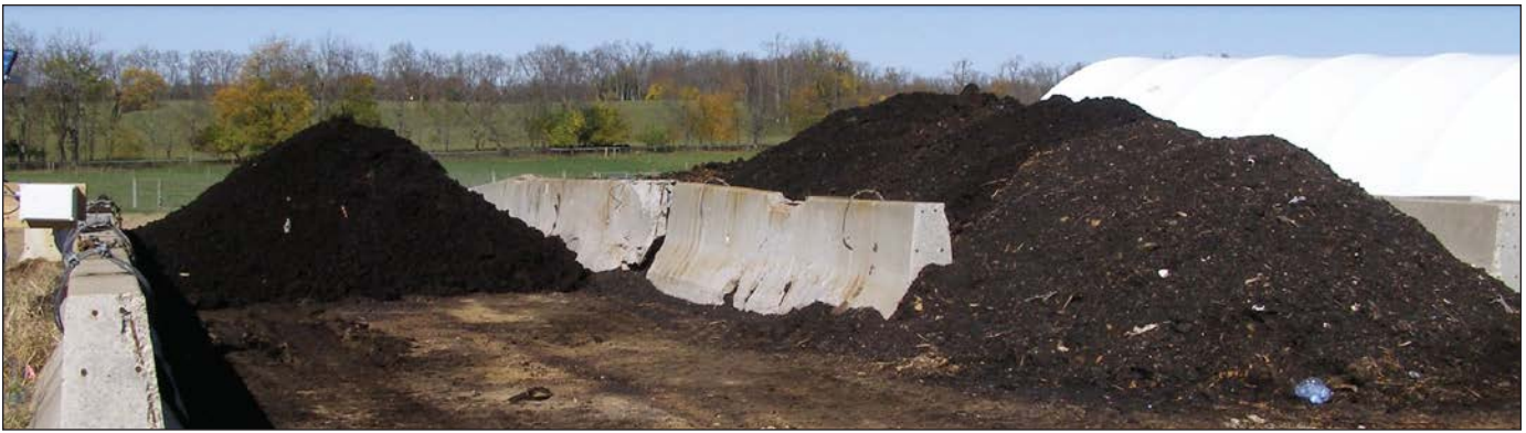
Figure 4. Example of a bin composting system constructed using soil cement flooring and construction barriers.
