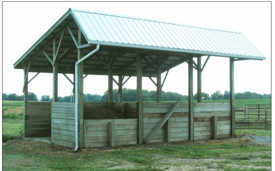
Figure 5. A three-bin shed with roof and doors.
