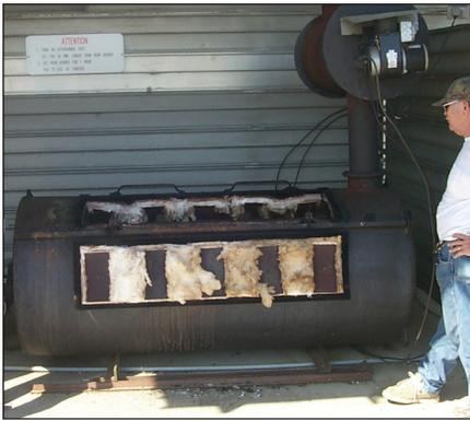
**Figure 1.** An example of an incinerator with an afterburner.
